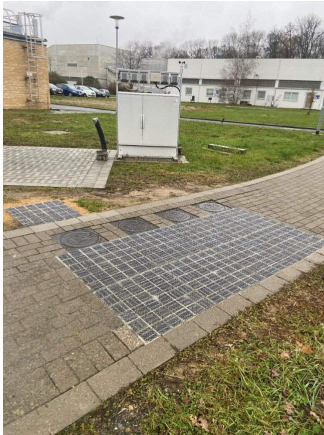
Figure 2.3 The RIPV pilot project Silicon Crystallin modules in Julich - Germany
